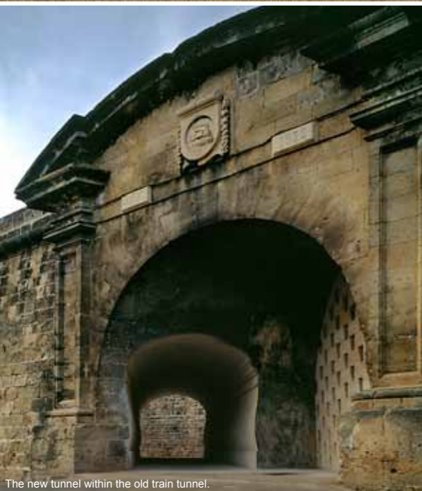
The new tunnel within the old train tunnel.
