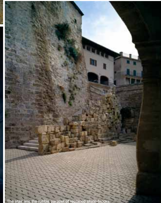
The stair and the rubble parapet of replaced stone-blocks.
